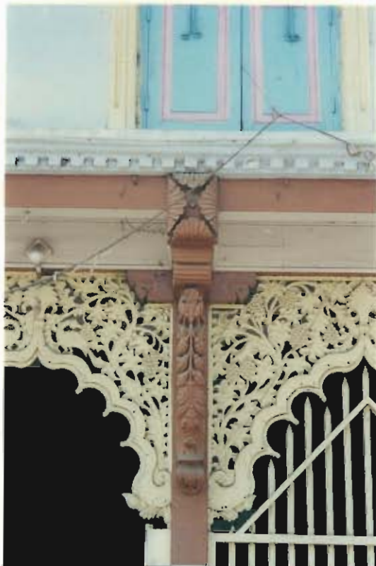
View of a carved timber arch in the Front elevation
