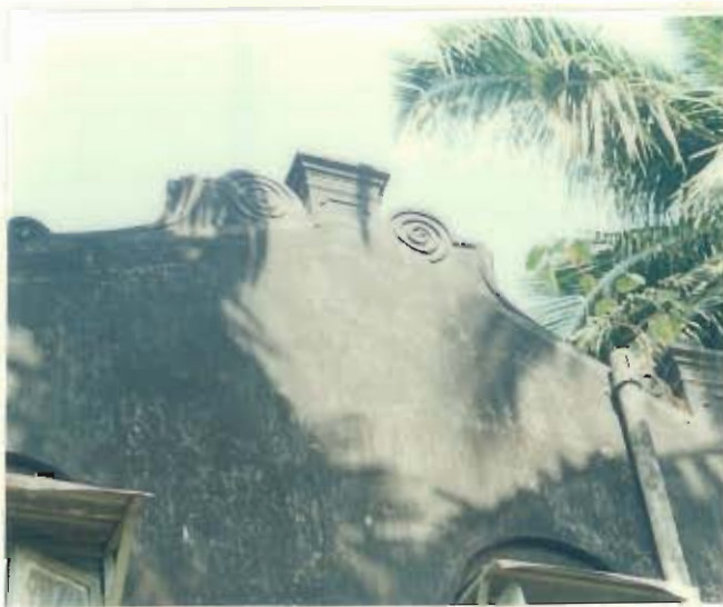
View of the rear gable wall of the church
