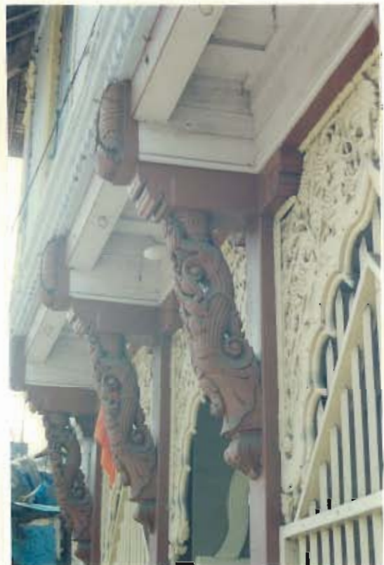
View the carved timber bracket supporting Projection of upper floor
