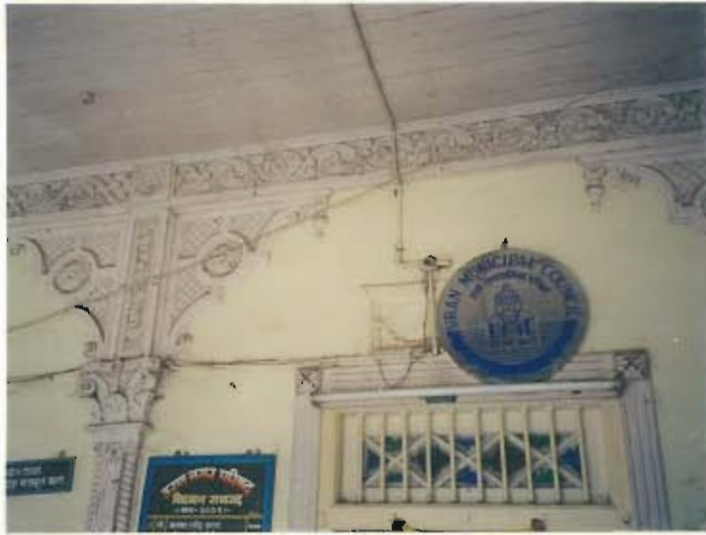
Rich timber carvings in timber moldings mounted on the walls and timber carving strip along the timber ceiling in the verandah
