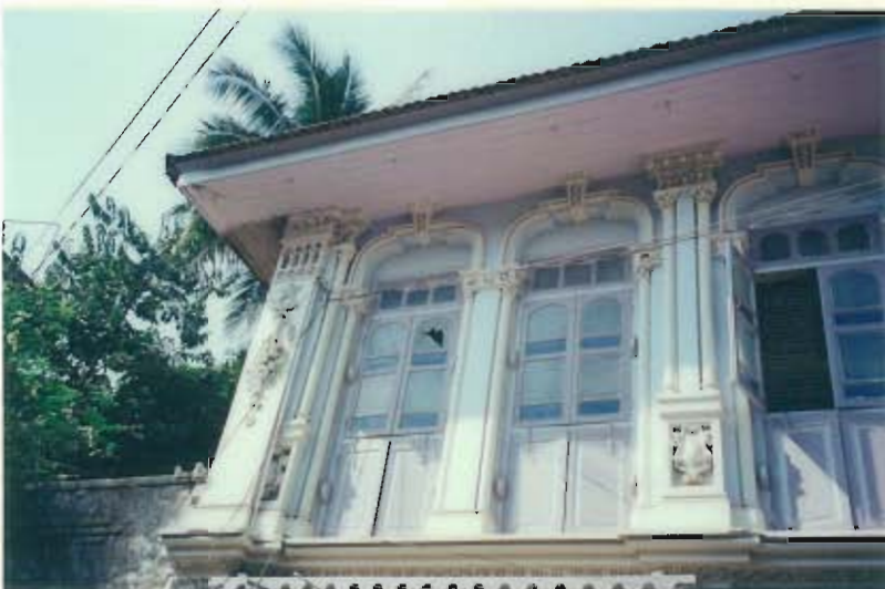
Baroque style stucco details seen on upper floor of the house facing road
