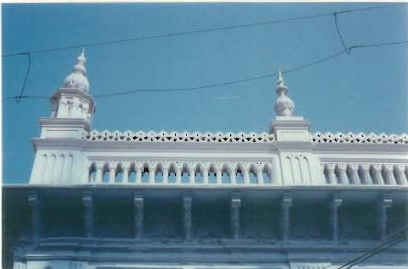
Details showing parapet, Chajja and brackets of the prayer hall of Mosque
