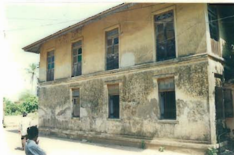
Side elevation of the school building
