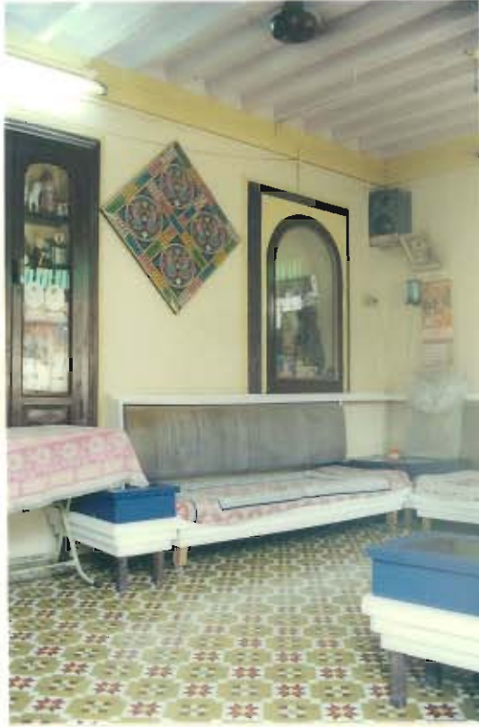
View of living hall on first floor showing patterned floor tiles and timber joist roofing with timber boarding
