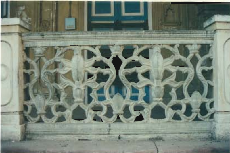
View of typical pre fabricated railing panel With delicate details.
