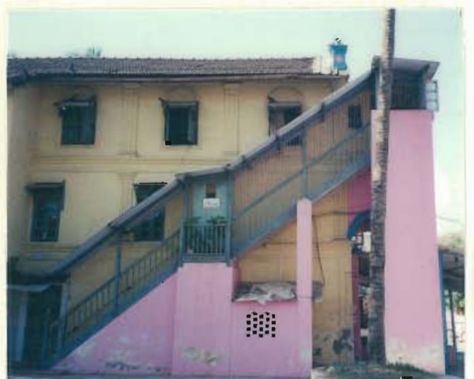
View of the external staircase on the eastern side
