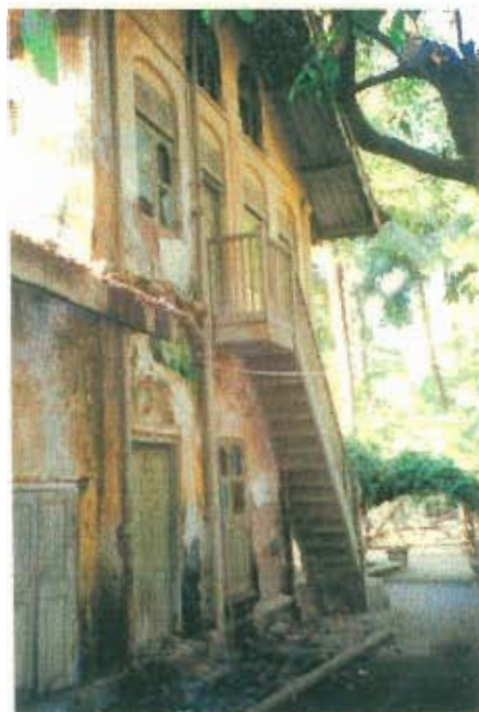
View of the north east corner of the structure
