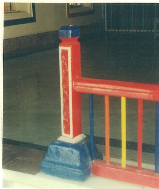
View of the timber railing in the sabhamandapa
