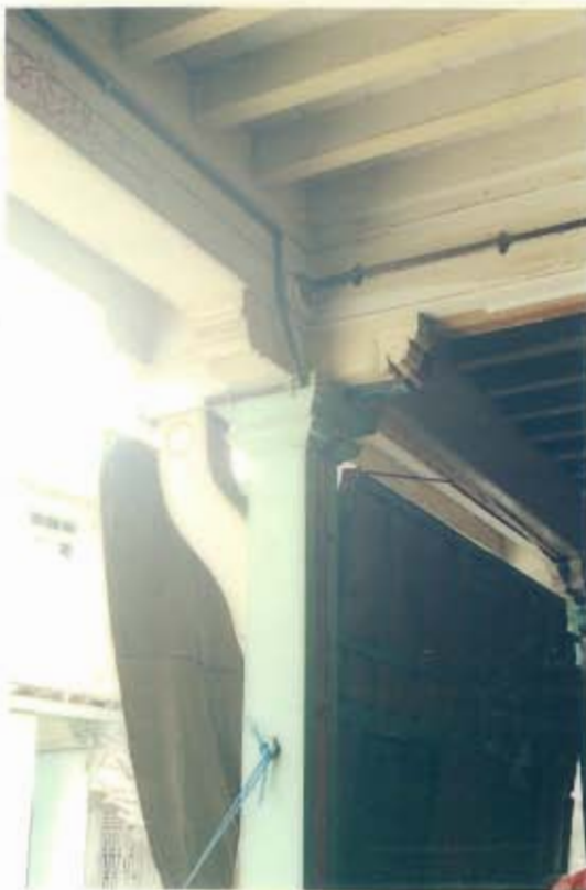
View of a typical bracket supporting with Projected beam with above
