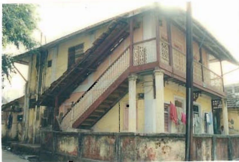
View of external staircase from corner of street
