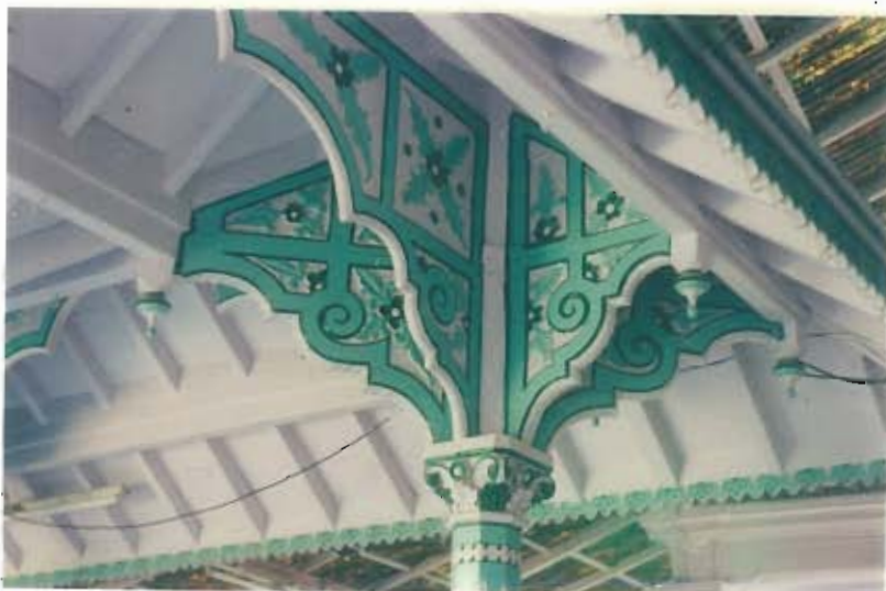
Details showing timber bracket supporting roof in the ablution tank
