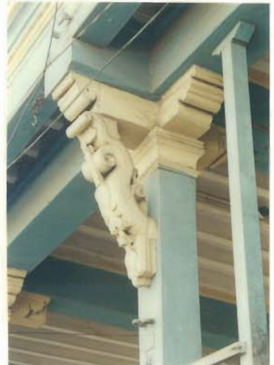
View of the articulated timber bracket
