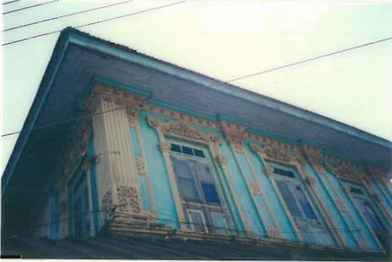
View of details showing Baroque style stucco details on upper floor
