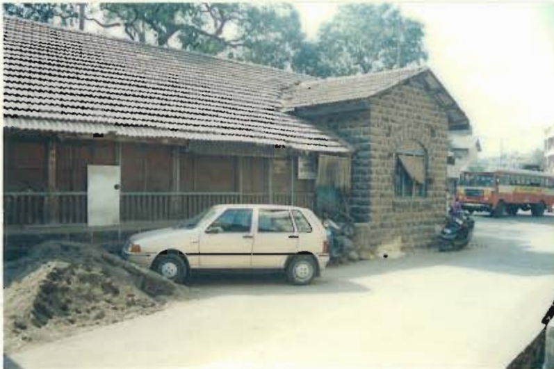
View from Wani Aali shows covered verandah with timber partition
