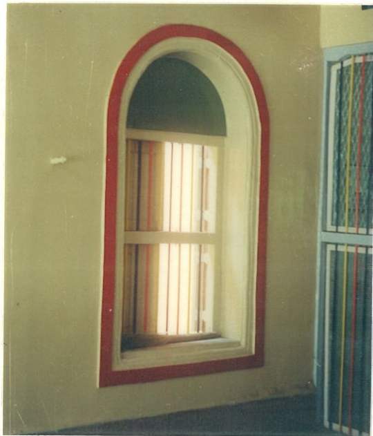
View of the typical window in Sabhamandapa
