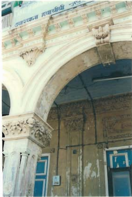
View of details showing decorative stucco work on arch and masonry column.
