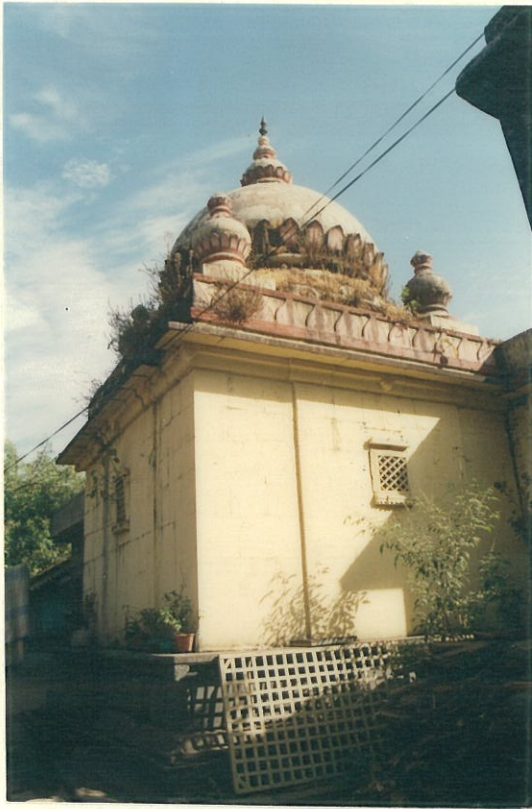
View of Dome and Garbhagriha From south
